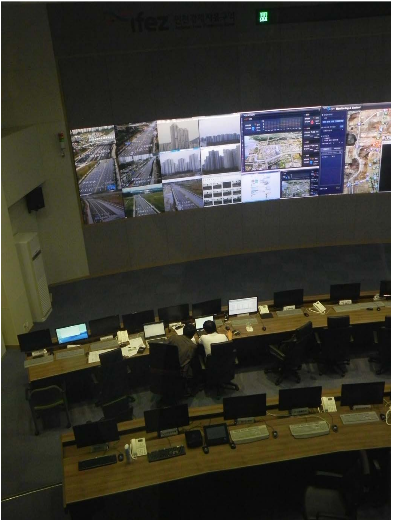
Figure 5. Songdo Control Room, September 2, 2013
